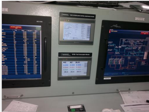
ETNP-10 and EFCM monitors in ECR. Main units installed in consoles.
