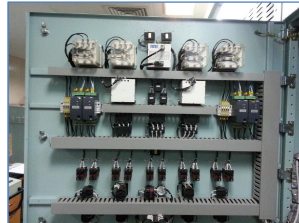
EPM after installation
