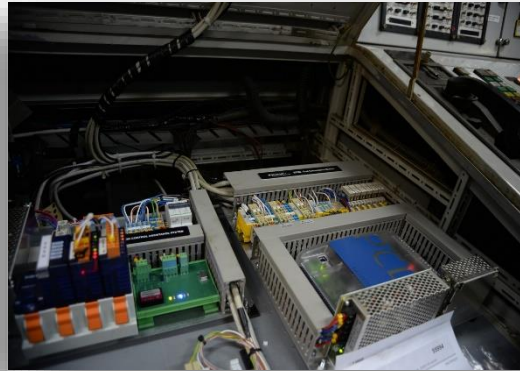
ETNP-10 and EFCM monitors in ECR. Main units installed in consoles.
