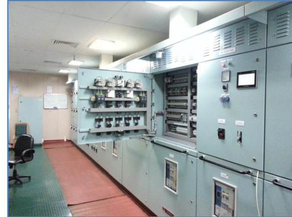
EPM during installation
